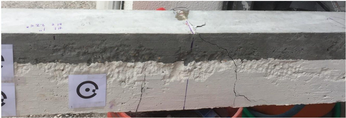
Figure 4-3 Shear Flexure Cracking
